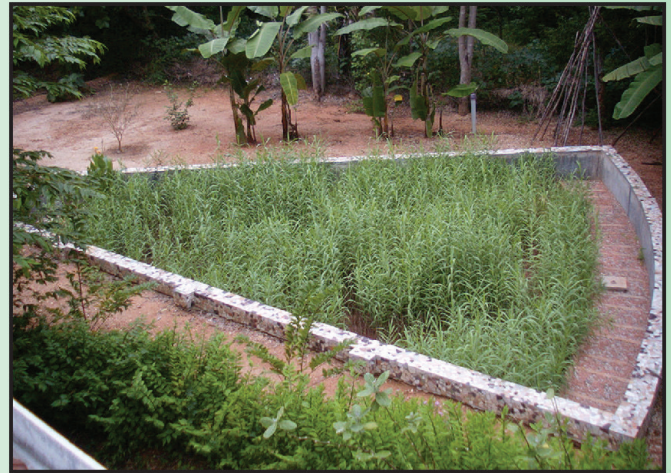
Rootzone treatment system for domestic wastewater reuse for irrigation in operation since 1994 in Auroville Township, Tamil Nadu, India.
