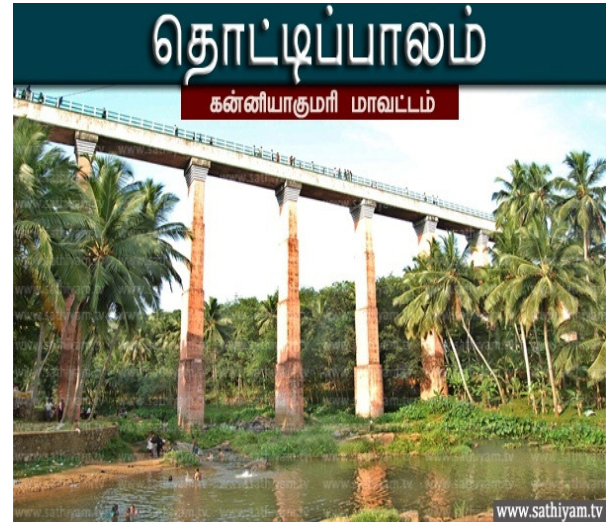
Mathoor Hanging Bridge
